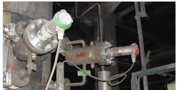
Trimod Besta level switch type: HAA 22C01 041 Besta float chamber type: I021-1C0RC1
