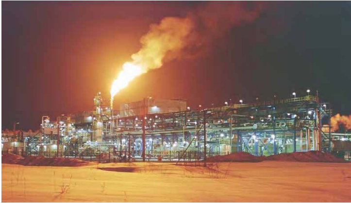
Source: Luginetsky Gas Compressor Station Strezhevoy, Western Siberia, Russia
